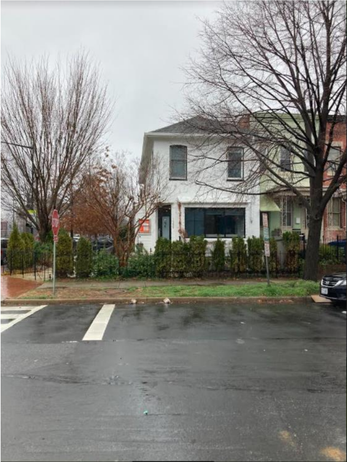
Photo Number 1: D Street Frontage
